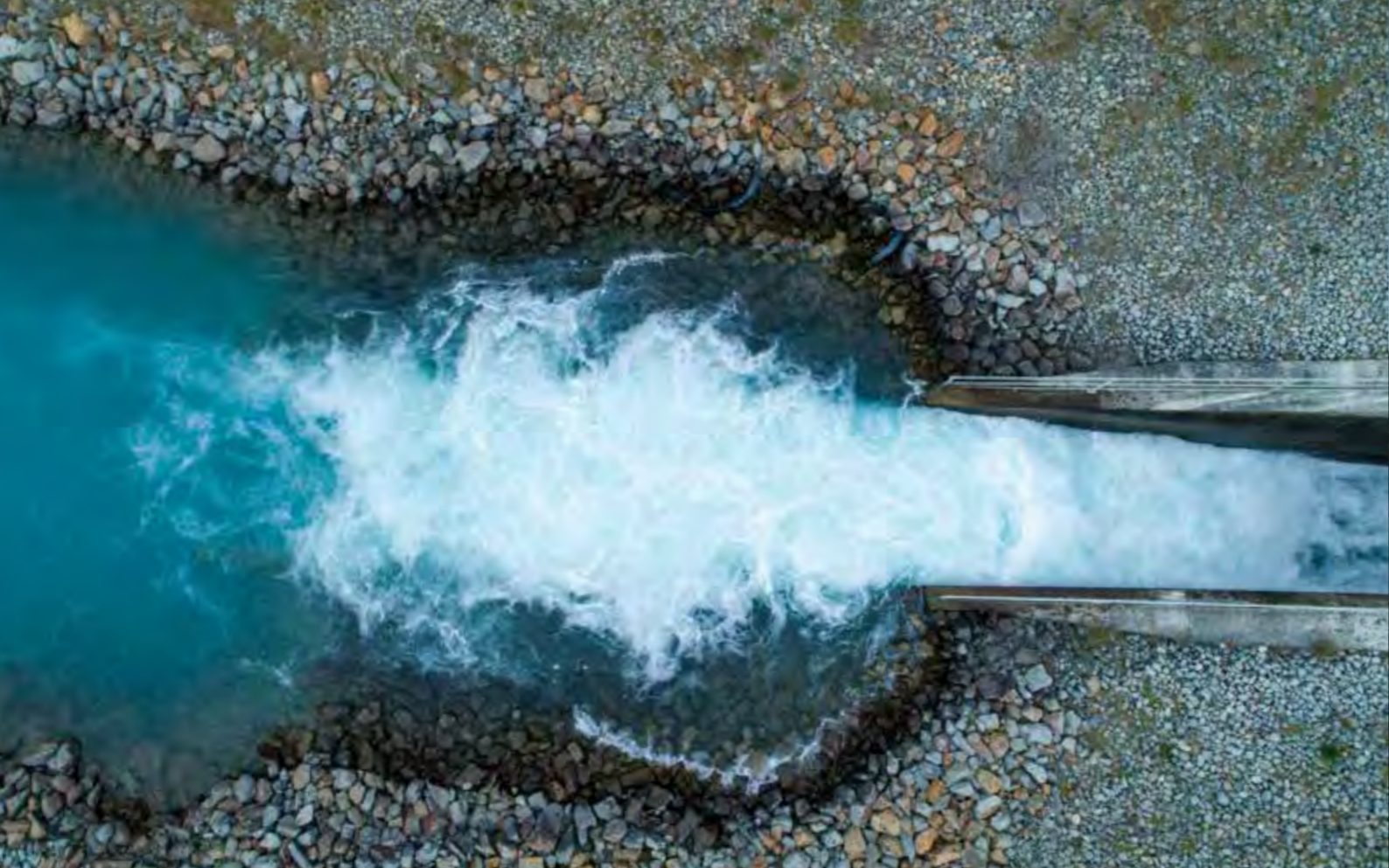
Rakaia headrace control gate.
