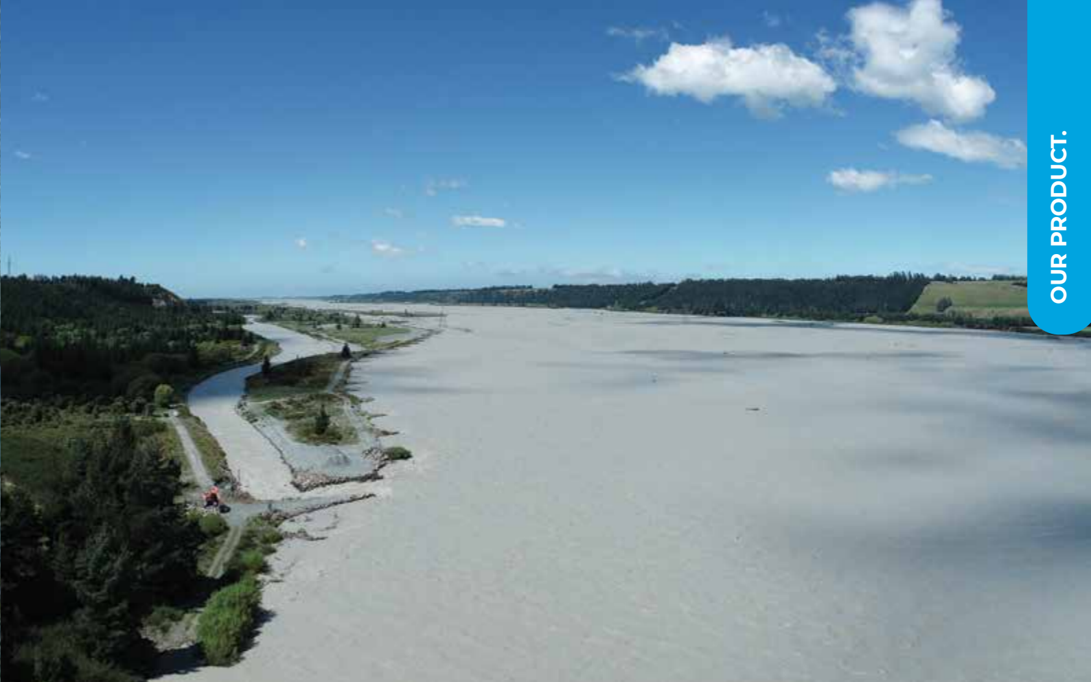
Flooding at Rakaia intake point.
